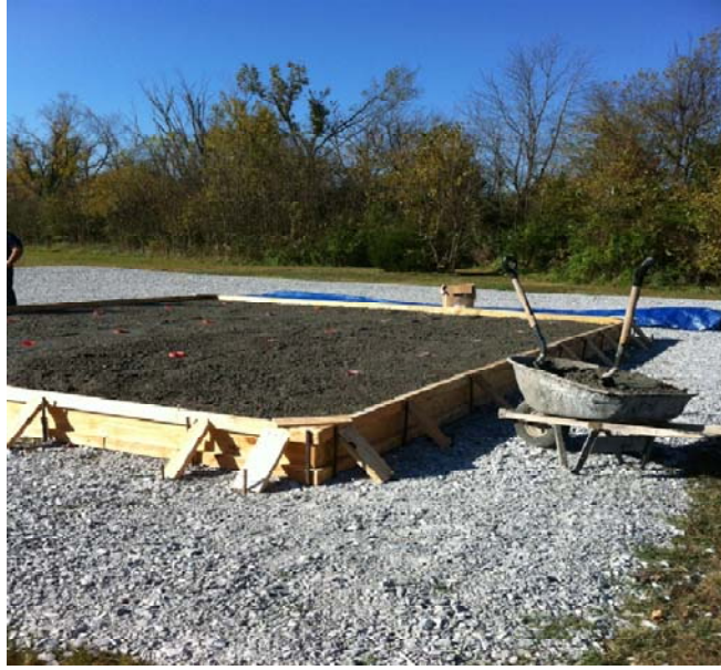
Figure 5.3: 24' x 20' 10" thick concrete base mat (Osweiler, 2012)
